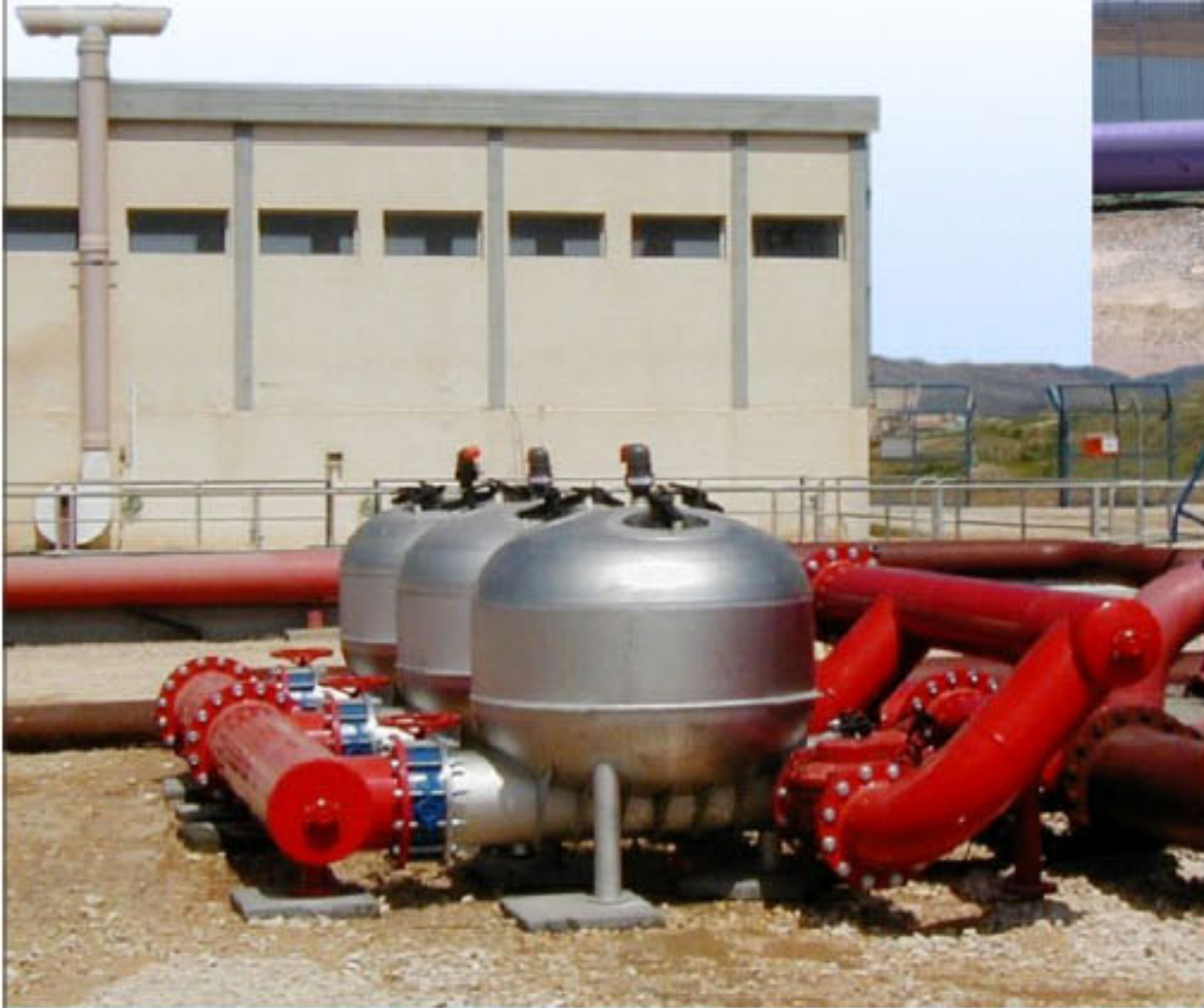
Waste water recycling for irrigation, Mekorot Ma'ale Kishon - Israel 1,600 m 3 /h, 200 micron (80 mesh)
