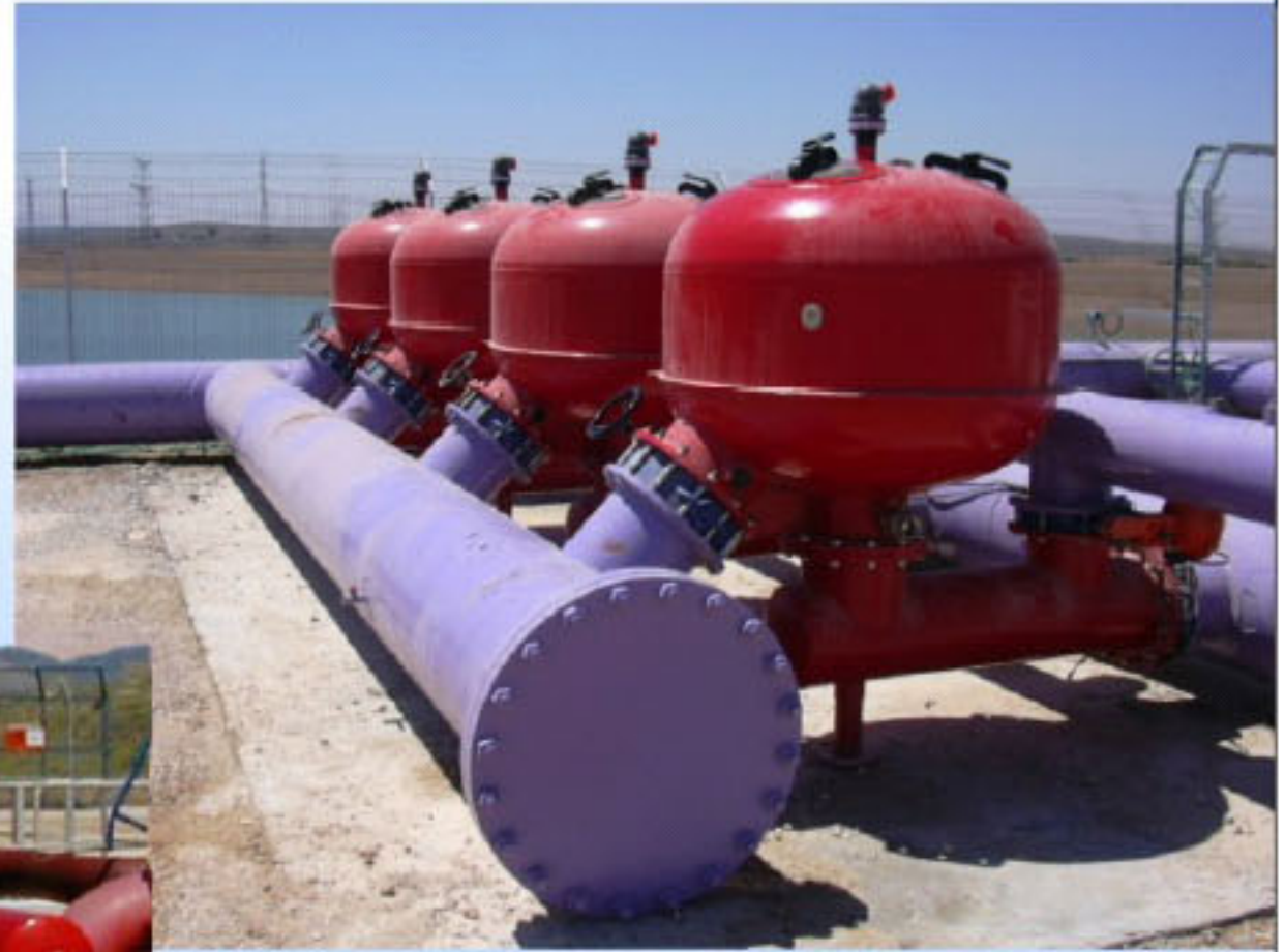
Jerusalem's waste water recycling for irrigation, Kfar Menachem - Israel 3,000 m 3 /h, 200 micron (80 mesh)
